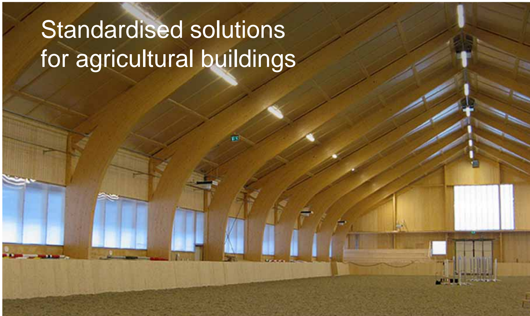
Finnforest Kerto, Glulam, roof elements Manege, Espoo, Finland
