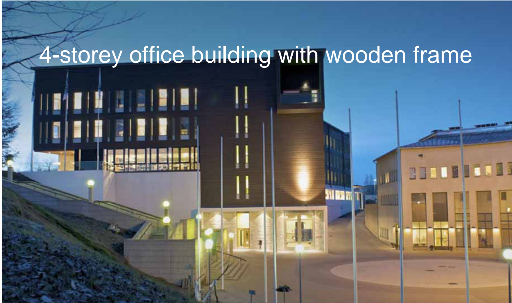
Finnforest Glulam frame, Finnforest Kerto intermediate floor elements Pilke House, Metsähallitus, Rovaniemi, Finland
