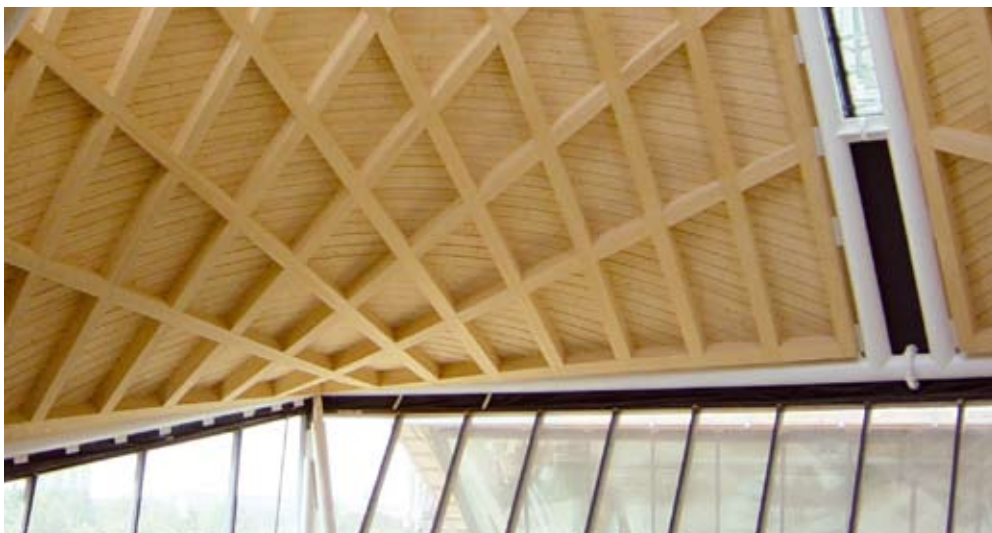
Lattice shell structure out of glued and screwed spruce lamellas.
