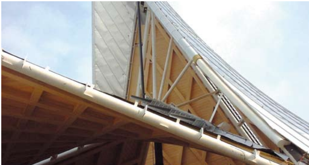
External view before glass is installed.
