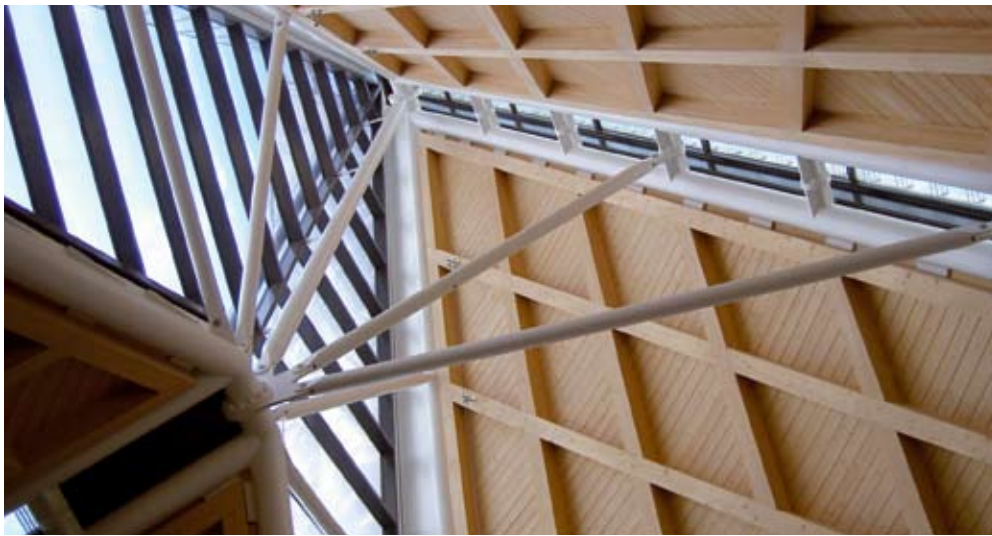
Interior view to the raise with timber structure and curtain walling.
